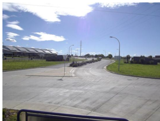
Figure 2.5: The Ringers Road (looking west)
